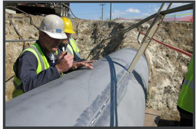
Present (Exposed Pipeline)
